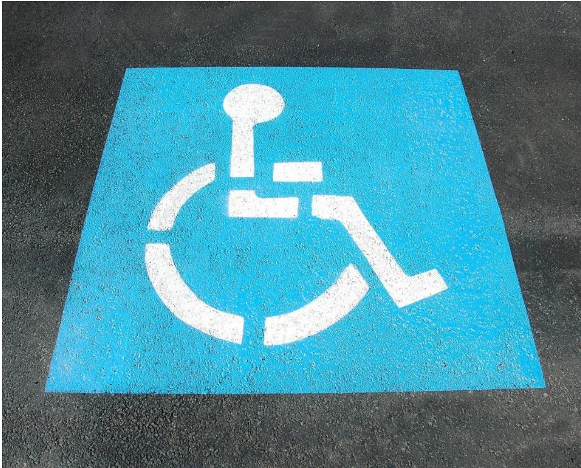
Figure 7. Disabled car parking space marking
